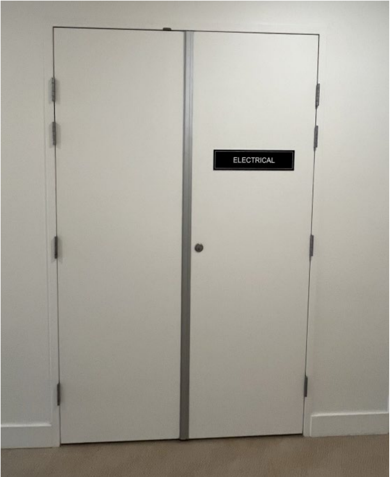
Image: An example of a utility cupboard in an apartment building
